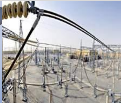
Grid sector Equipment & services for power transmission
